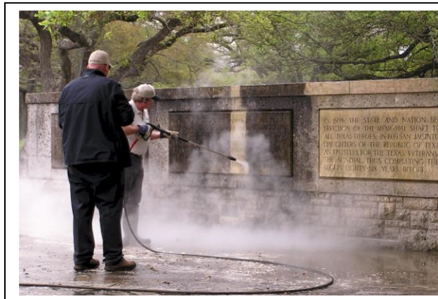
John Purswell and Bob Gruetzmacher cleaning the panels.
